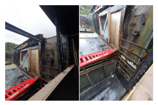
In areas where there is localised severe fire damage, the design team have recommended the removal of these roof sections with charred structural joists for health and safety reasons. They have also recommended the installation of waterproofing works to ensure areas that are in relatively good condition do not deteriorate. These works will be undertaken in the coming weeks and will reduce the scope of the main repair and reinstatement works.
